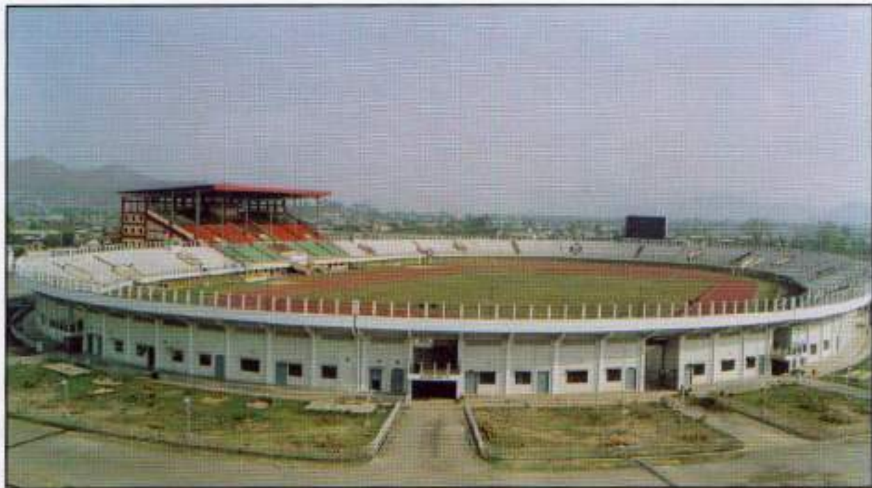
MAIN STADIUM KHUMAN LAMPAK SPORTS COMPLEX [ 25,000 CAPACITY GALLERY WITH 2,500 VIP ENCLOSURE 8-LANE, 400 M SYNTHETIC TRACK WITH PHOTOFINISH SYSTEM ]
